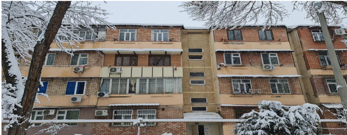
Fig. 2. The actual condition of the building at the time of the experiment.
